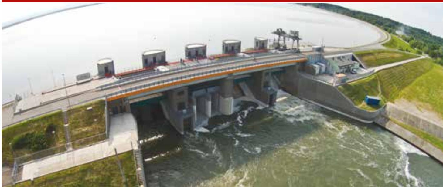
Flood preventing measures included modernising the existing retention basins and building new ones, modernising the dam and pump-room in Zwierzyniec, side dam and pump-room in Siestrzechowice as well as building a road bridge, service buildings on a dam in Nysa, building fish passes and modernising the technology.
